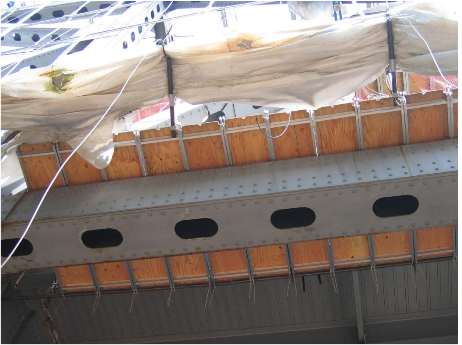
Aluma Beam Support System, Plywood Flooring, & End Containment System
