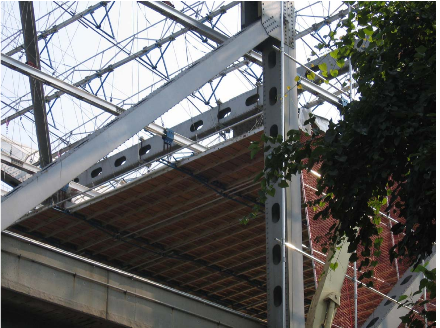
Rolling Truss, Putlog, & Aluma Beam Framing System w/Plywood Floor
