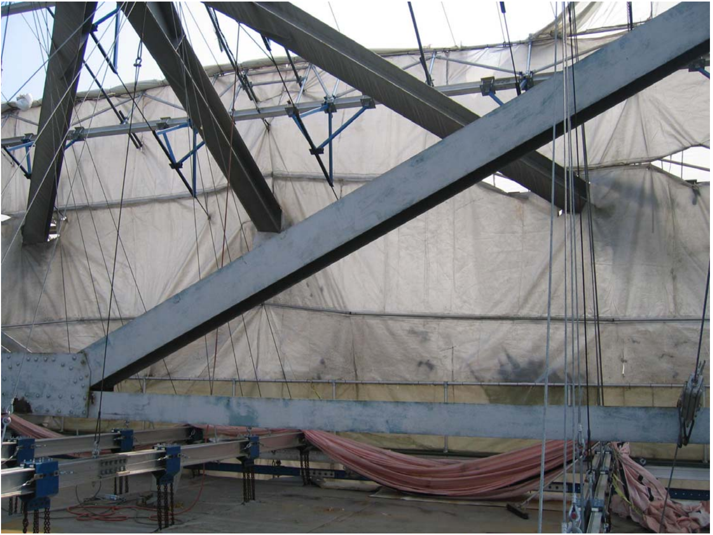
Aluma Beam Trolley Supports Vertical Trolley Supports & Containment Tarpaulins
