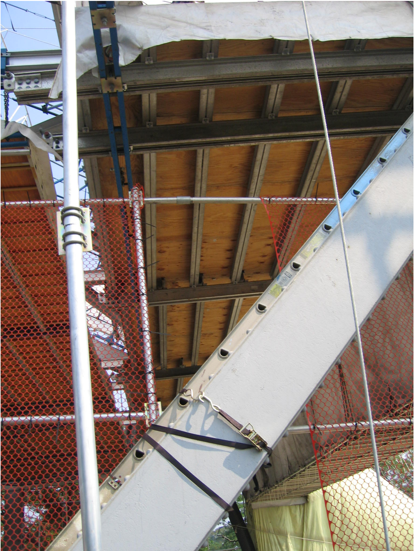
Aluma Beam Support System, Plywood Flooring, Side & End Containment System
