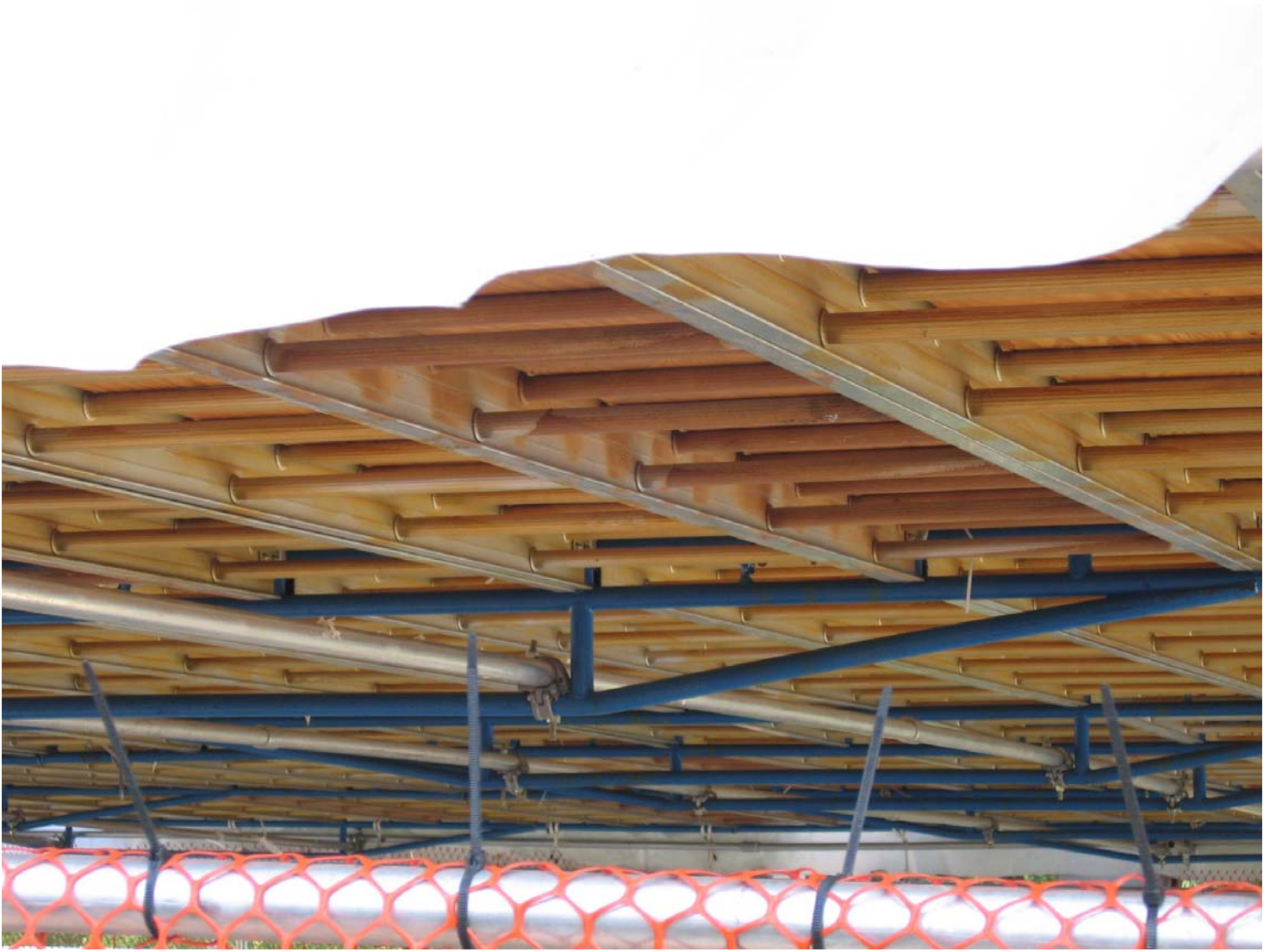
Aluma Beam Put Log Support System & Plywood Flooring
