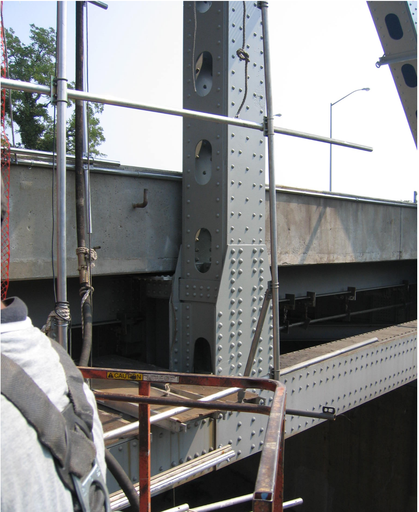
Tube & Hanger Scaffold system for Containment Support
