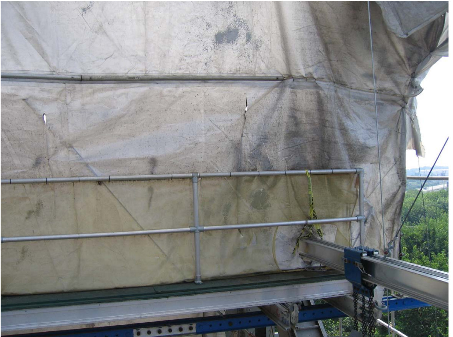
Containment Tarpaulins, Trolley Support, Handrail & Aluma Beam Framing
