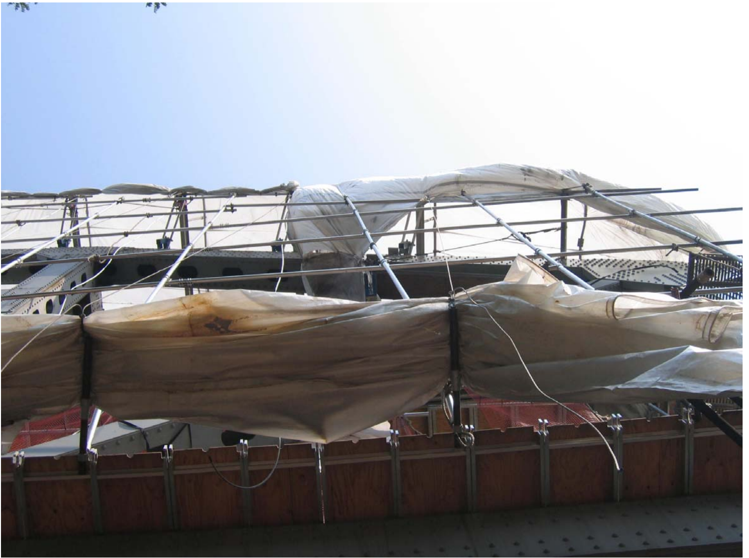
Aluma Beam Support System, Plywood Flooring, & Side Containment Framing System
