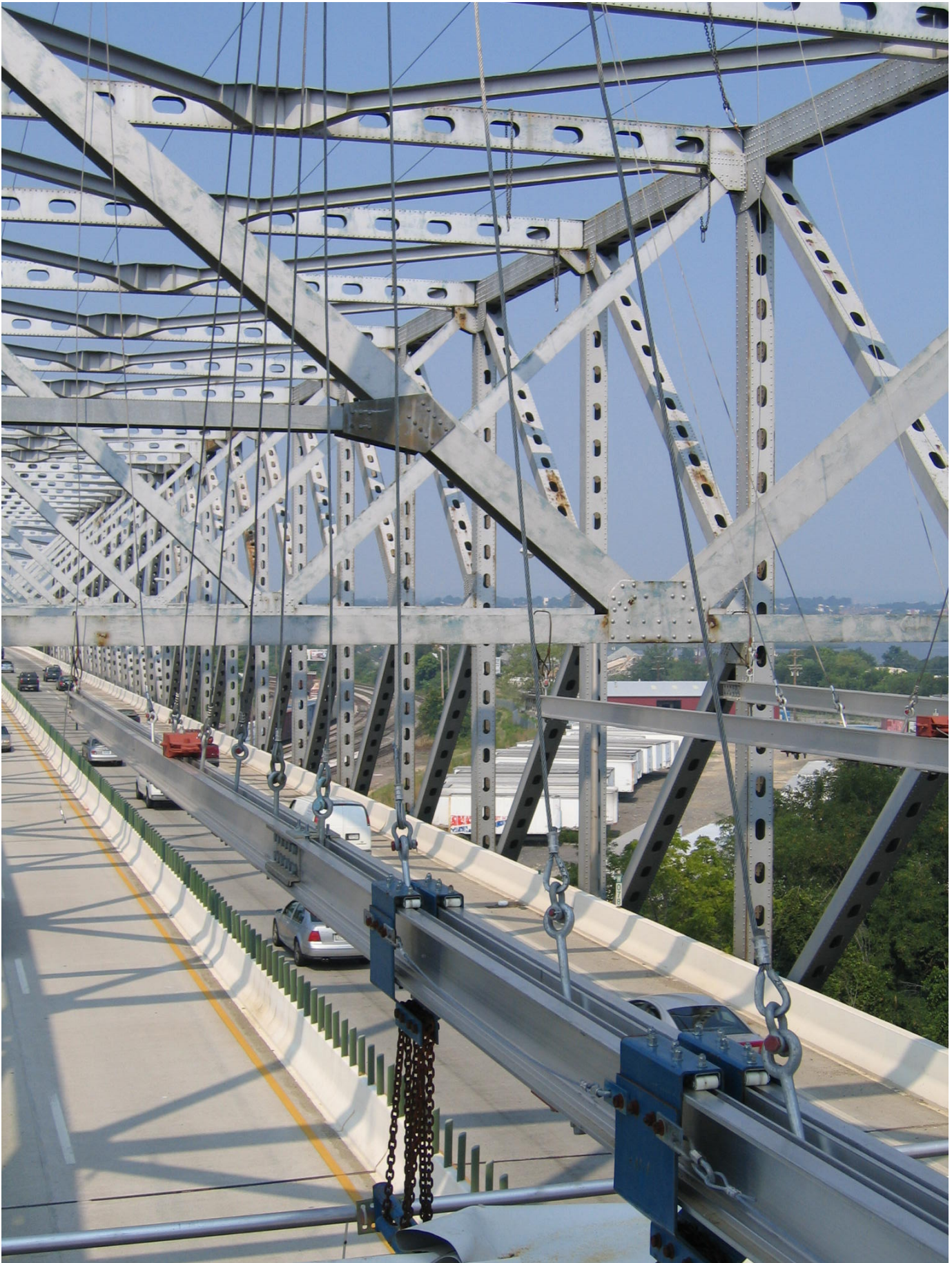
Aluma Beam Framing Trolley Supports & Vertical Tie Up Supports
