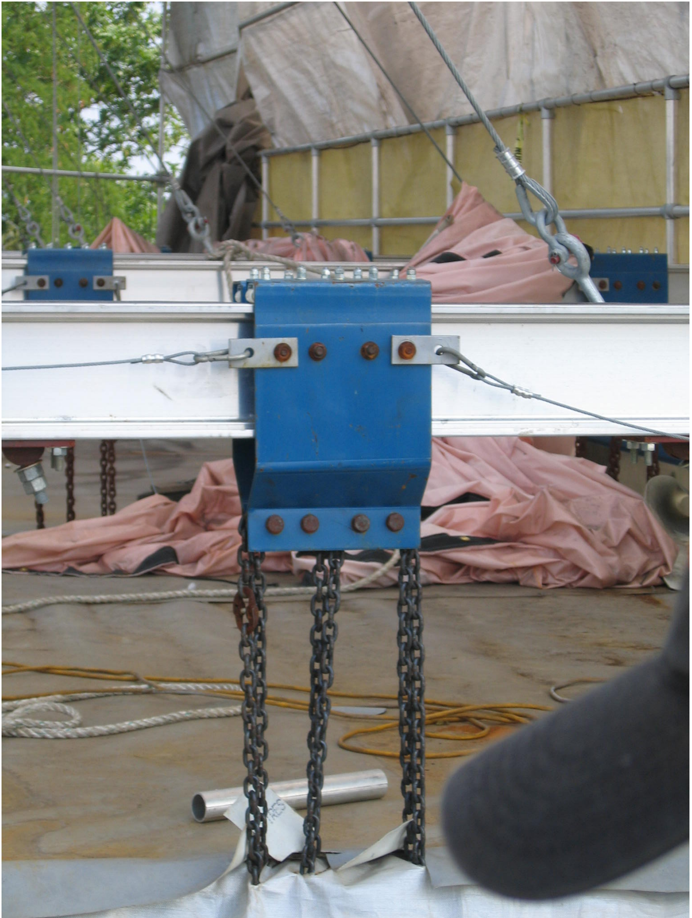
Platform Support Trolley, Containment and Floor System
