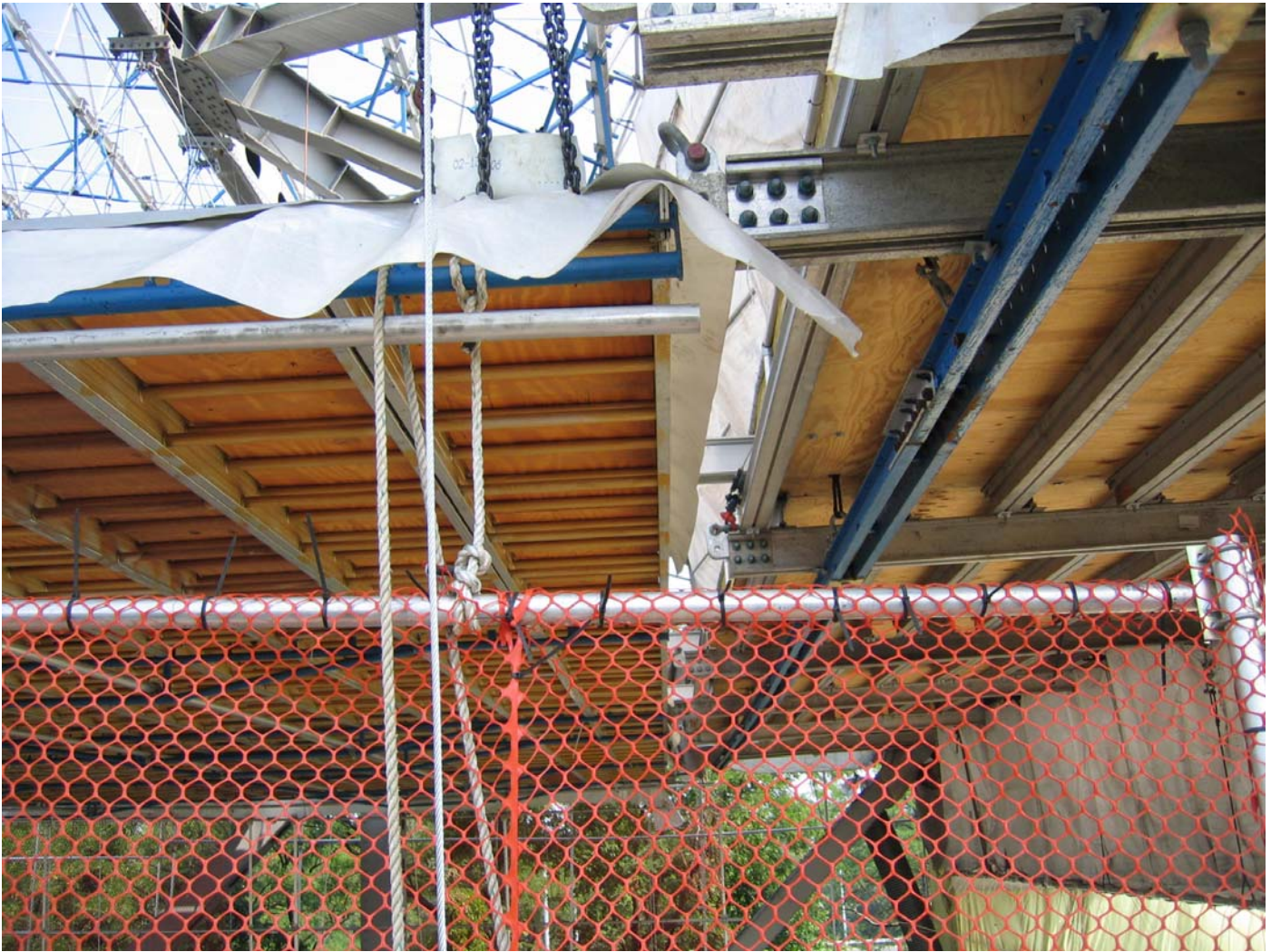
Aluma Beam Support System & Plywood Flooring
