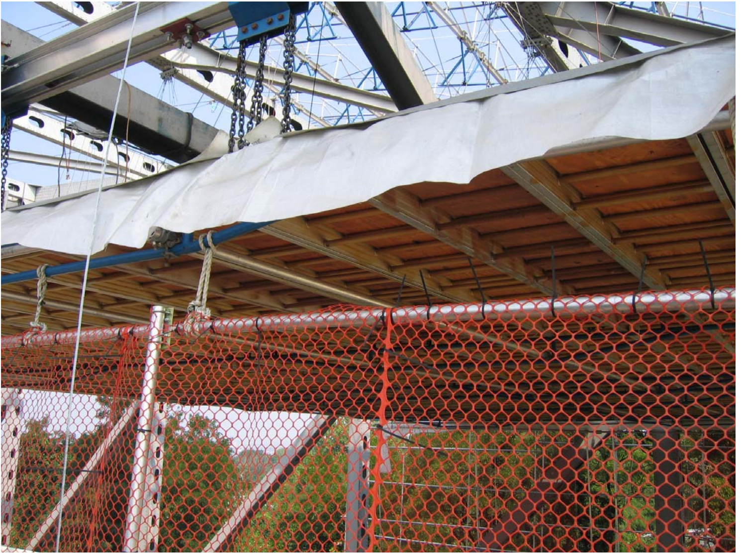
Aluma Beam Support System & Plywood Flooring
