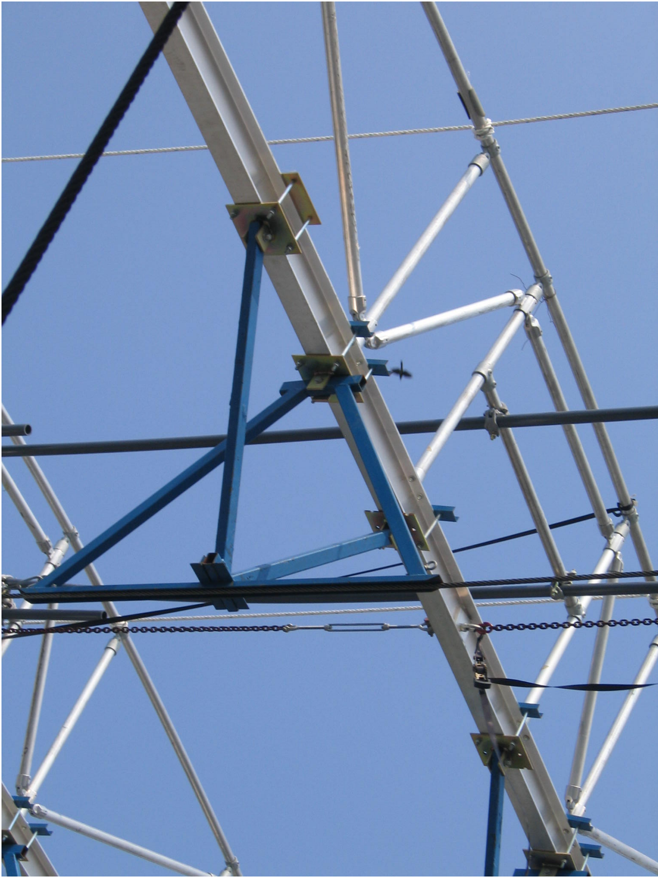
Upper Truss Chord Put Log Frames & Containment Scaffolding Support
