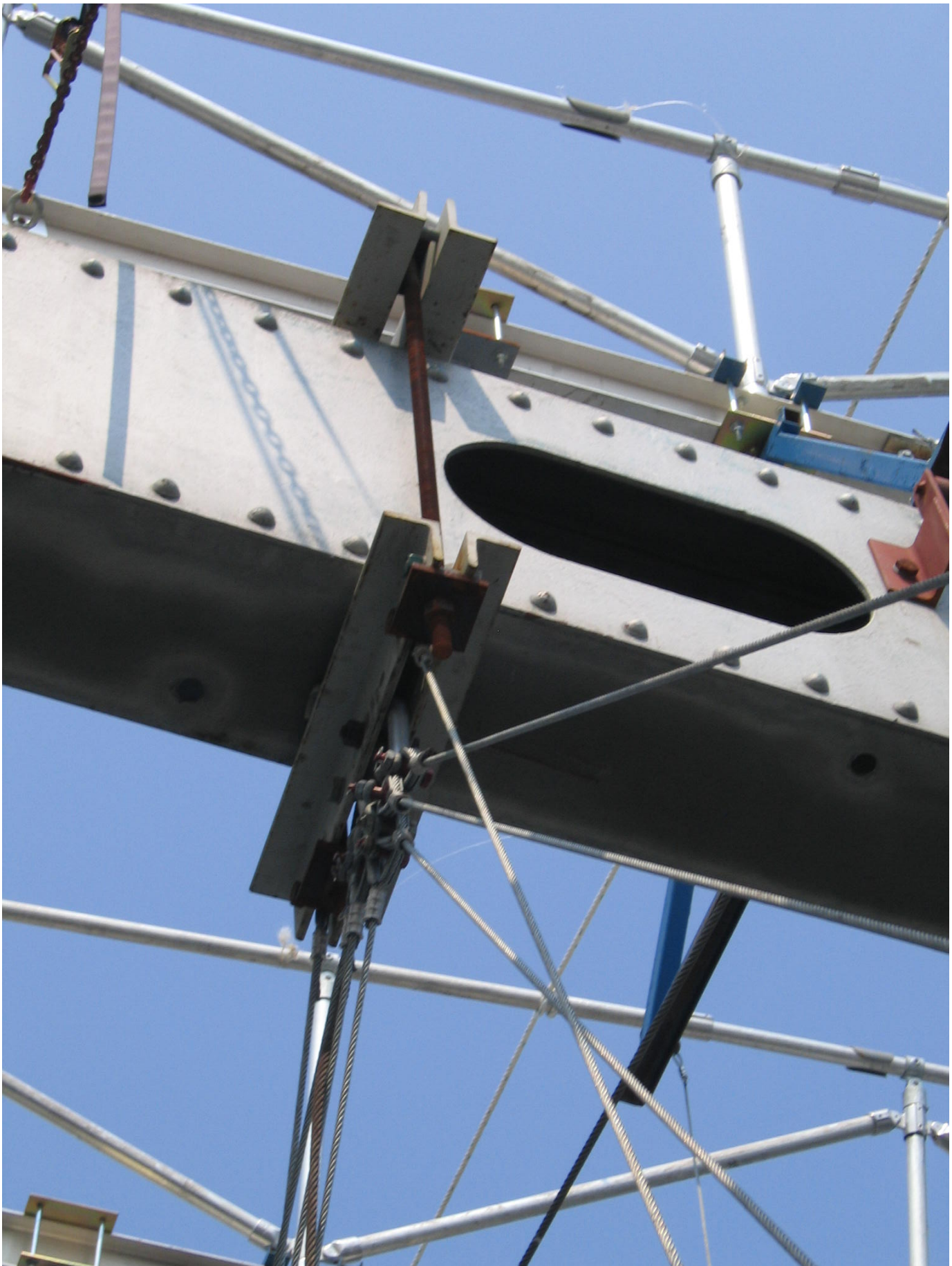
Upper Truss Chord Support Assembly
