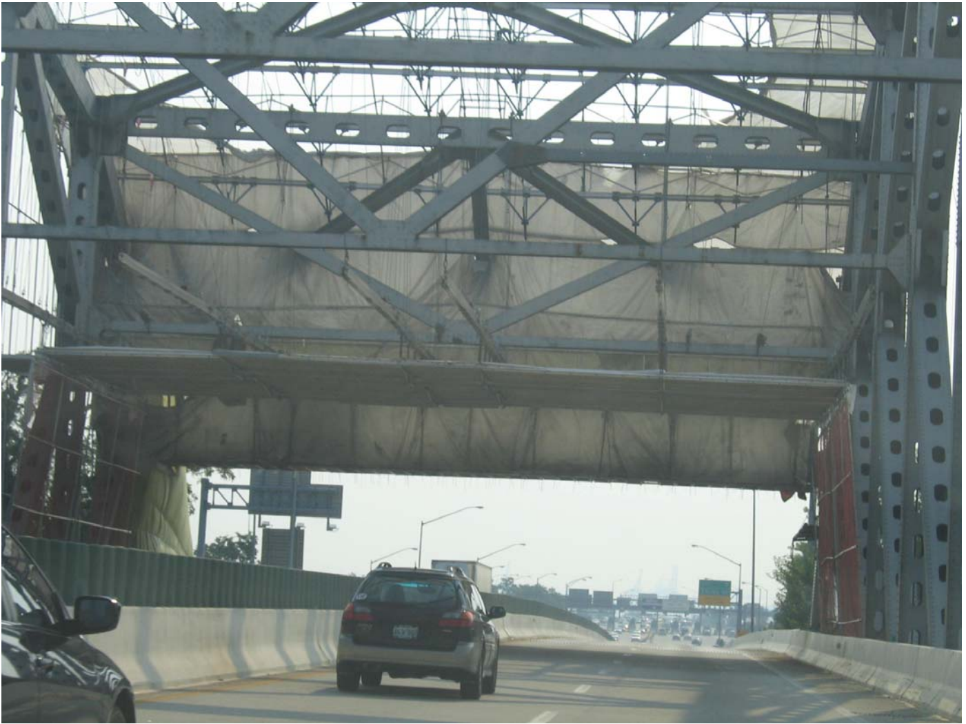
Upper Truss Chord Supported Rolling Platform & Containment Platform Below Roadway
