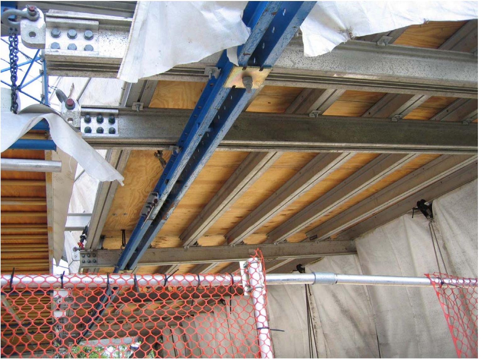
Aluma Beam Support System & Plywood Flooring
