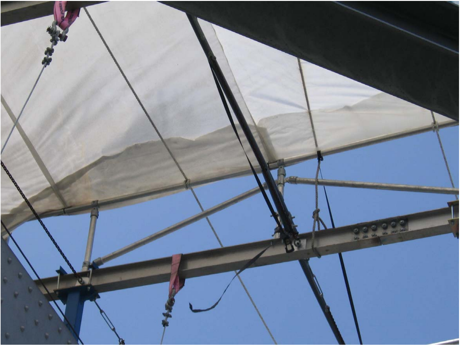
Upper Containment Tarpaulins
