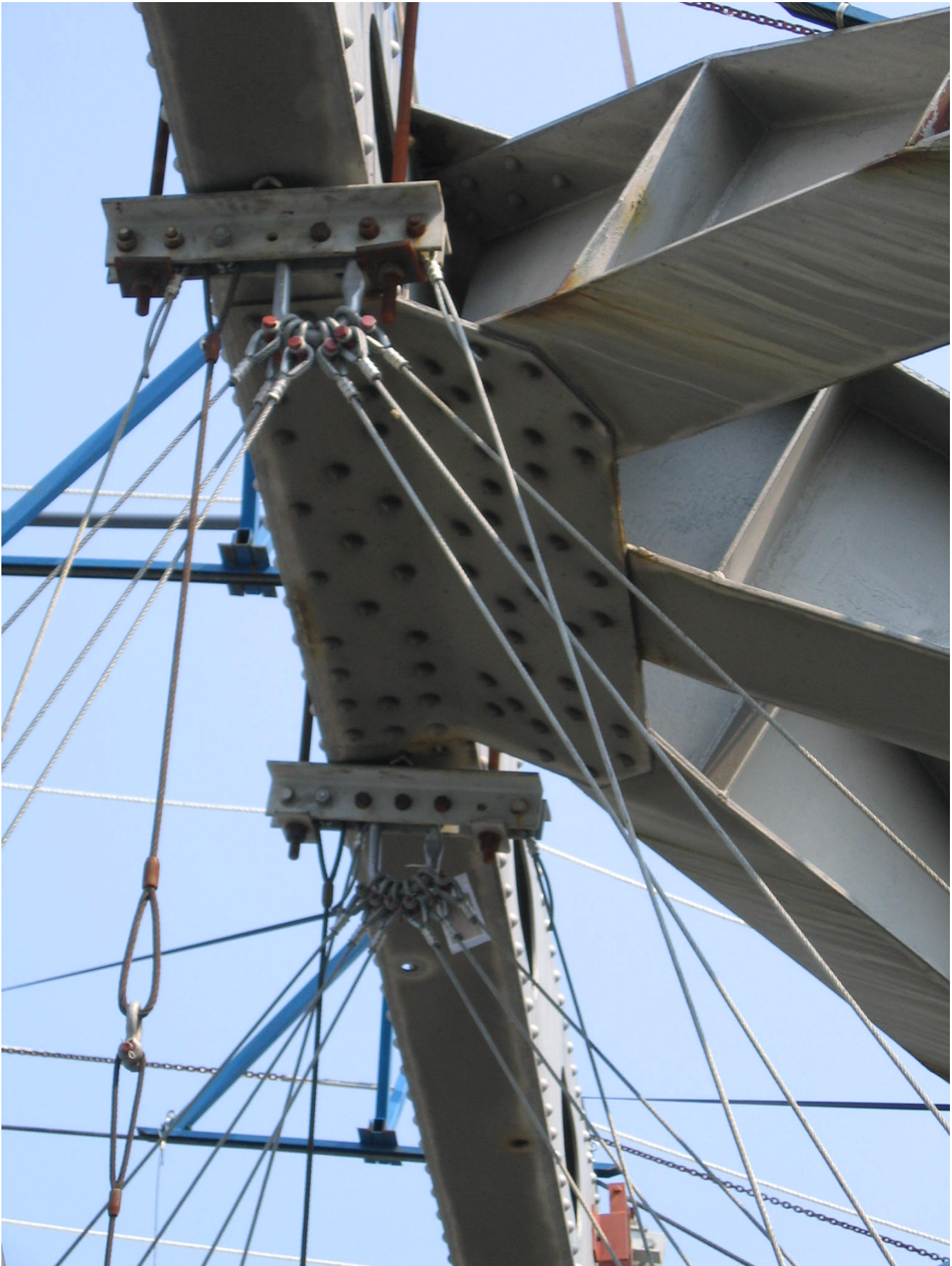
Upper Truss Chord Support Assemblies
